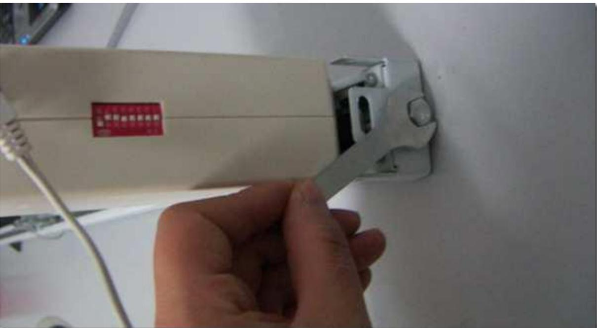
15. Install the tracks to your preferable position with the wall brackets or ceiling brackets. Then attach the track on the brackets slots.
