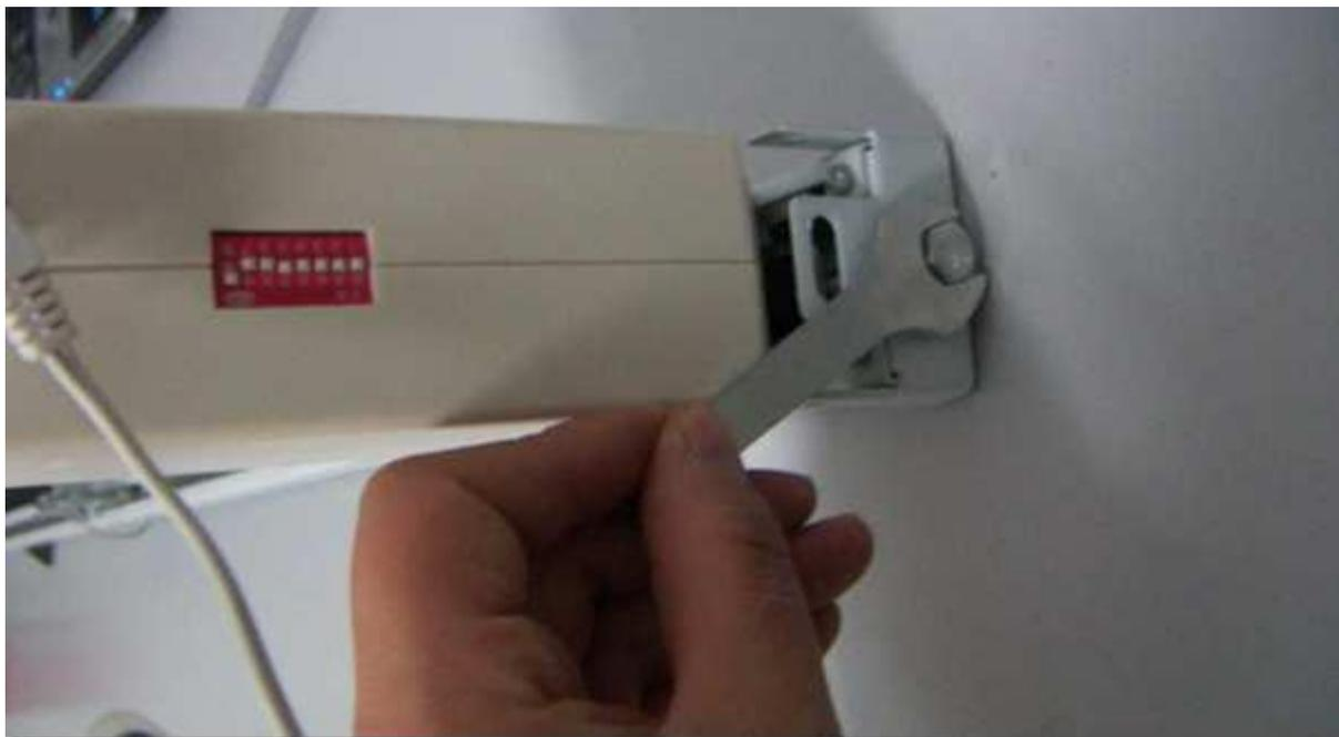
10. Pull back the steel wire as tight as possible and fasten the big-head screw with a screwdriver. Make sure the steel wire still separately stays on their side.
